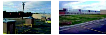
BNSF's remediation sheds are gone, MDC lines are underground, parking areas are landscaped and approximately 6,600 square feet of property will be available in the future for new commercial construction.
