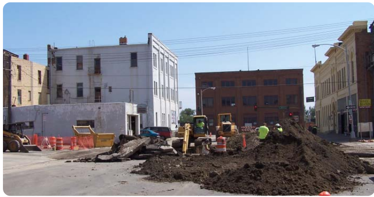
Trenching has been necessary in downtown Mandan to install pipelines to connect a series of extraction wells to remediation gathering and treatment facilities. The Mandan Remediation Trust, the N.D. Health Department, the Mandan City Commission and LBG thank businesses, residents and visitors for your patience with the process.
