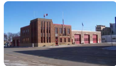
The Zone 2 satellite remediation building took the form of an addition to the Fire Station where it eventually will be used as a third bay.
