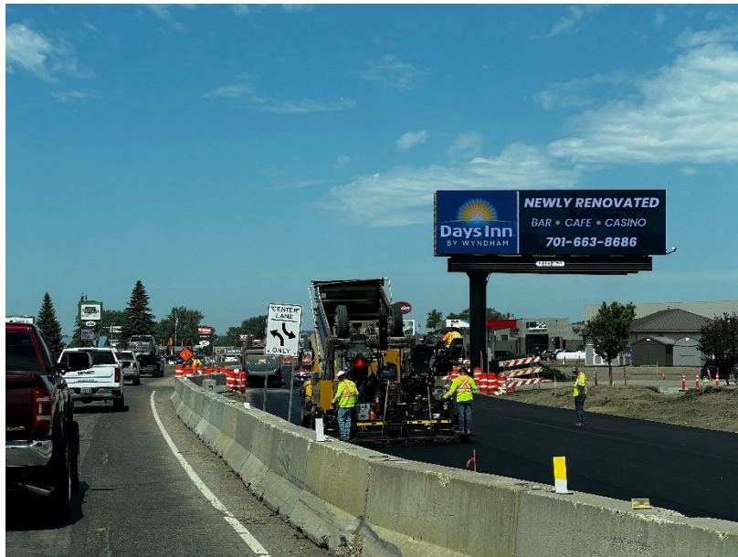
Photo of construction crew paving temporary road, taken in July 2025.
